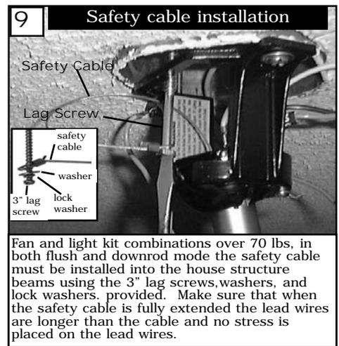
Fan and light kit combinations over 70 lbs, in both flush and downrod mode the safety cable must be installed into the house structure beams using the 3" lag screws, washers, and lock washers, provided. Make sure that when the safety cable is fully extended the lead wires are longer than the cable and no stress is placed on the lead wires.
